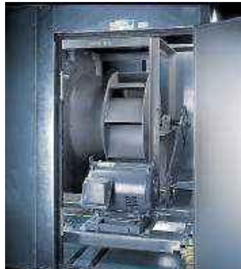
Figure 7: Plenum Fan
