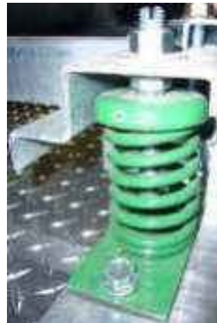
Figure 9: Spring Isolation
